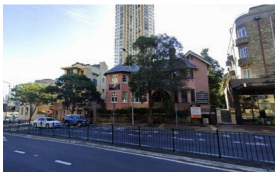
Existing Interface along New South Head Road
